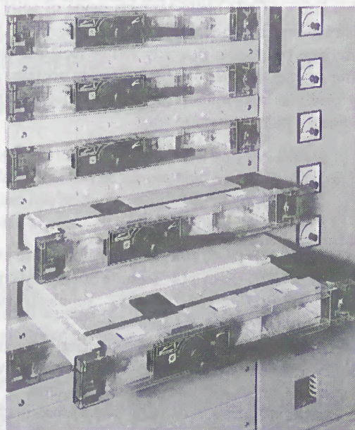
Fig. 8 - Industrial switchboard with switch-disconnector-fuses
