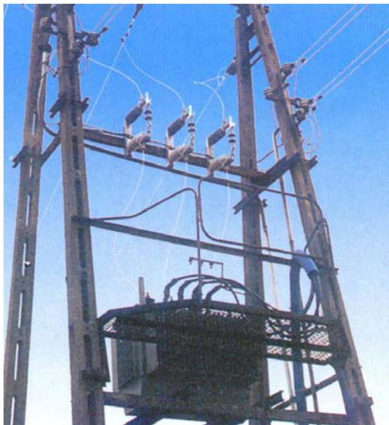
Fig.6 Combined short circuit current and overvoltage protection of an overhead transformer- distribution station using the High Voltage Protective Assembly type WZZ 17.5
