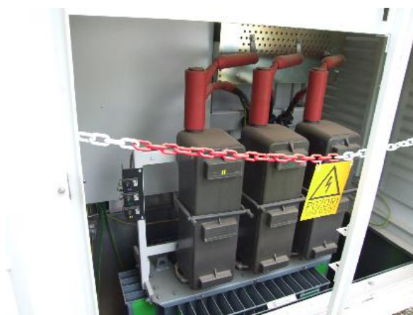
Figure 14: An example of application of fuse holder type VOH1, which insulates the HV part in a transformer substation
