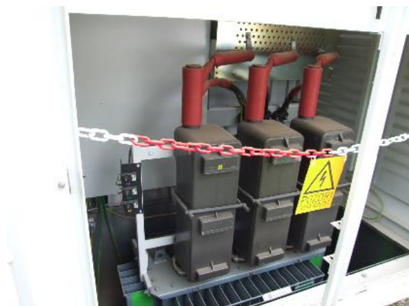
Figure 7: Fuse holder type VOH01 with elements for installation
